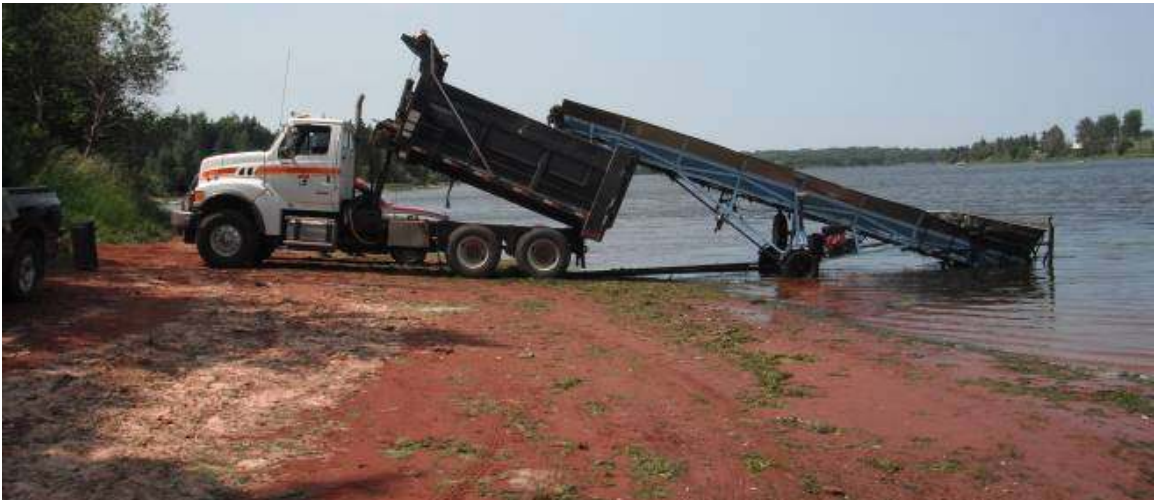
Figure 2. Shore conveyor and truck.
