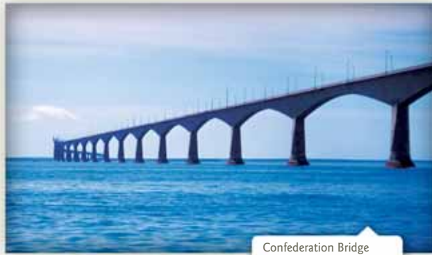
Confederation Bridge Photo by BRIAN MCINNIS
